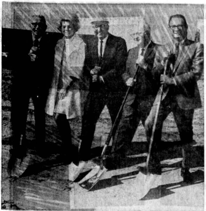
START WAREHOUSE... Construction is now underway in the city's Central Manufacturing District on a new warehouse for Wallich's Music City.
