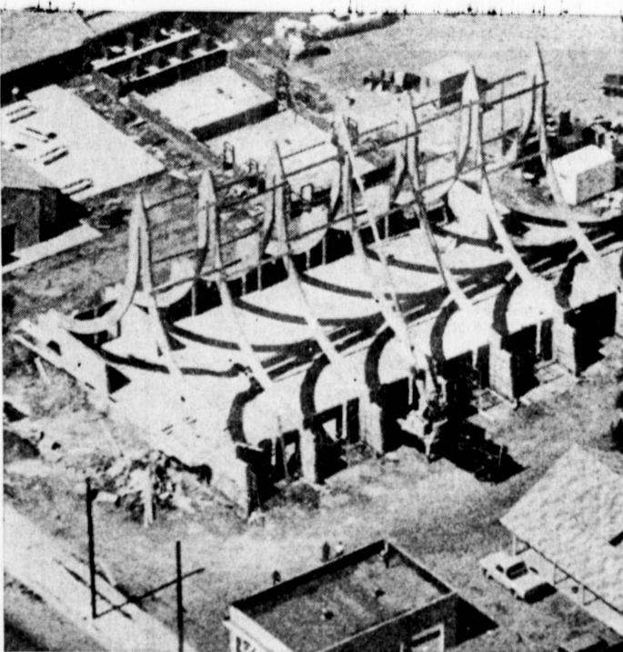
CHURCH RISES . . . This aerial photograph of Ascension Lutheran Church shows current building progress on the sanctuary, located at 17910 S. Prairie Ave. Members and Friends gathered Sunday for a cornerstone laying ceremony at the 450-seat structure. The inverted-arch laminated rafters symbolize praying hands. The Rev. Erwin Kurth, pastor of Christ Lutheran Church, Los Angeles, was guest speaker at the occasion.
