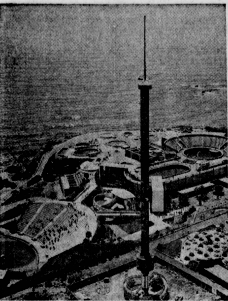
NEW LANDMARK . . . Marineland will dedicate a new California landmark Friday in ceremonies scheduled for 10 a.m. The $500,000 Sky Tower will take visitors to a height of 344 feet above sea level in a glass observation car which also rotates during the trip up and down a steel shaft. It will operate from 10 a.m. until sunset every day of the year.
