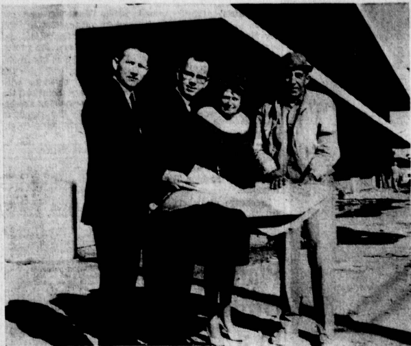
CHECKING PLANS . . . Supervisor Kenneth Hahn (second from left) and officials at Carson Elementary School examine plans for a new building at the school. With Hahn are, from left, Kenneth Miller, vice principal; Mrs. Minnie Wallace, and William Heiser, construction superintendent. The new building is scheduled for completion about April 15. Hahn was instrumental in speeding construction of the facility.
