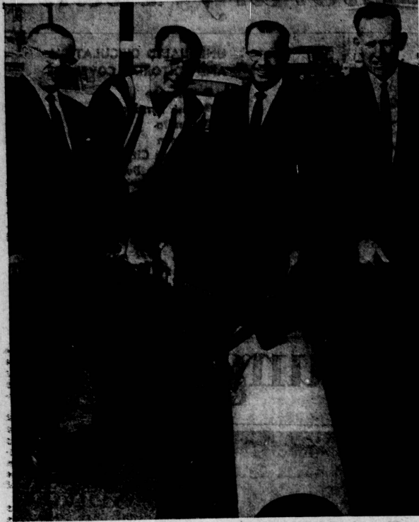
BEGIN PROJECT . . . Relocation of some 16,000 feet of 24-inch Dominguez Water Co. pipeline in Carson Street has begun. The first section of pipe is moved by (from left) R. B. Keith, president of the Carson Chamber of Commerce; Bert Lynn, a member of the Torrance School Board; Supervisor Kenneth Hahn, and Art Reeves, personnel director for the Water company. Movement of the pipe will make way for a long-planned improvement of Carson Street between Normandie and Figueroa streets.
