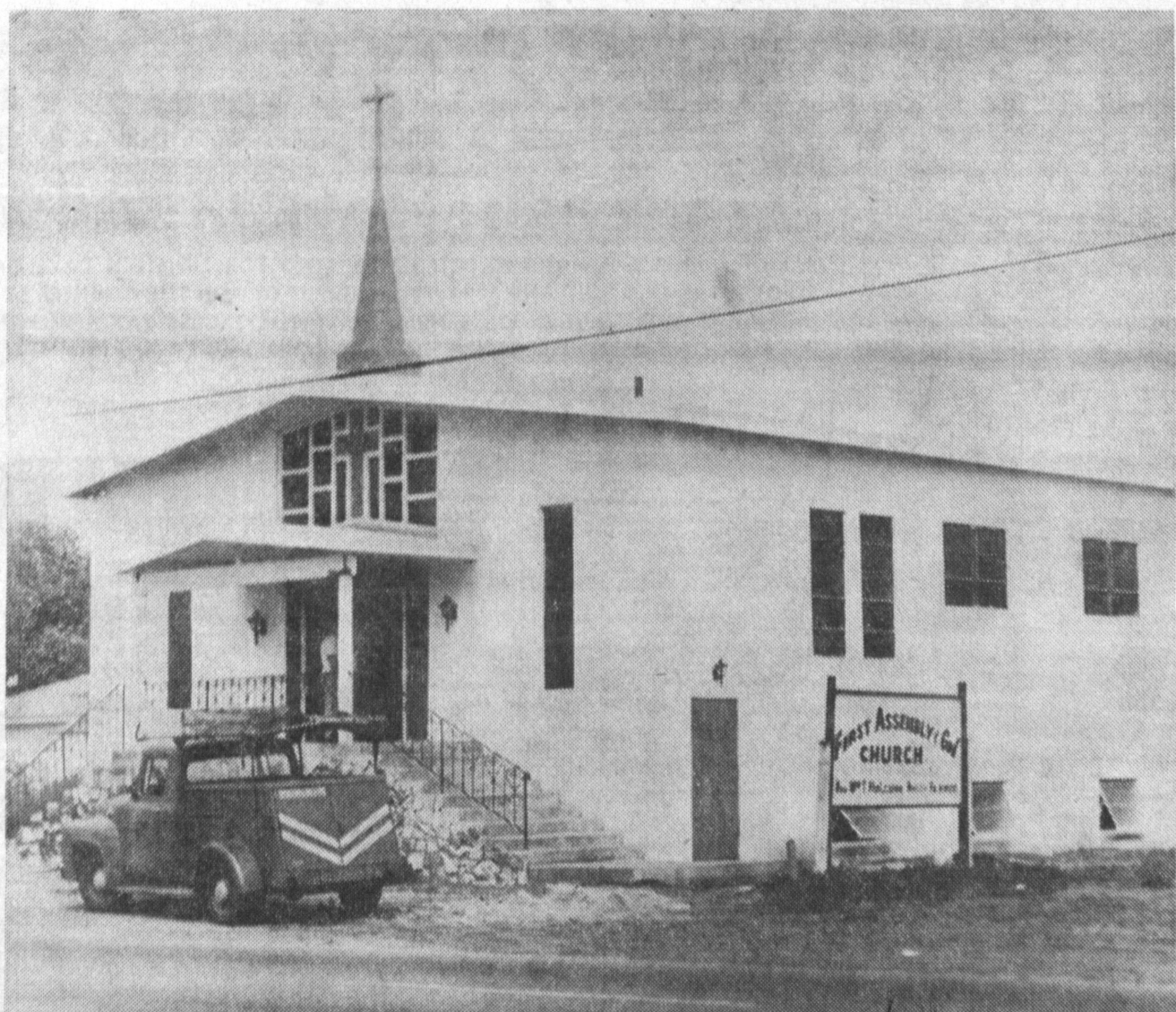
NEARING COMPLETION is the First Assembly of God Church located on Torrance Blvd. near Hawthorne Blvd. Members of the church have been
