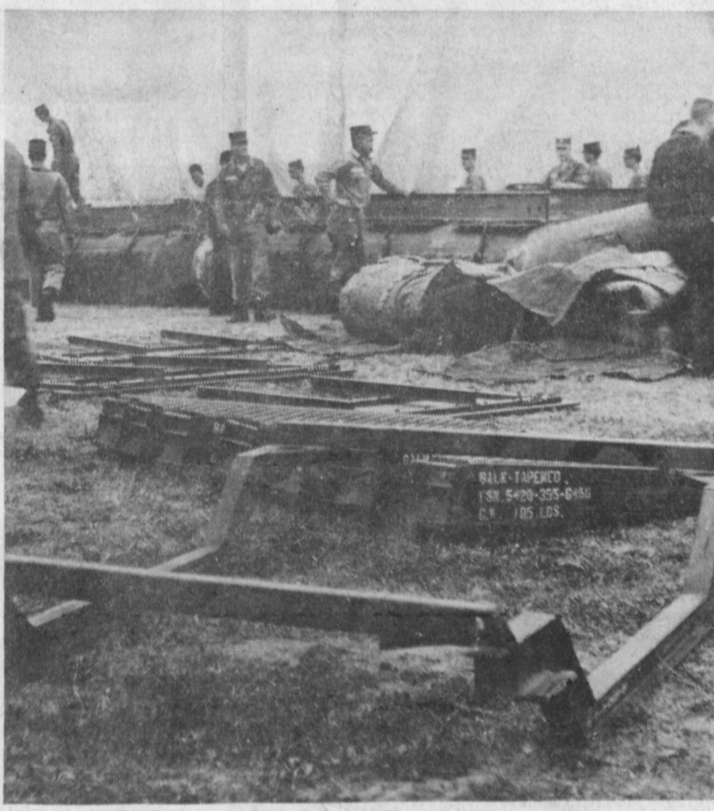
FLOATING BRIDGE erected for Armed Forces Day parade yesterday was being worked on late Friday by Company E 132nd Engineer Battalion, a special army bridge-building unit. The GIs worked Friday night to get their display ready for yesterday's combined services exhibitions at the Torrance Civic Center.
