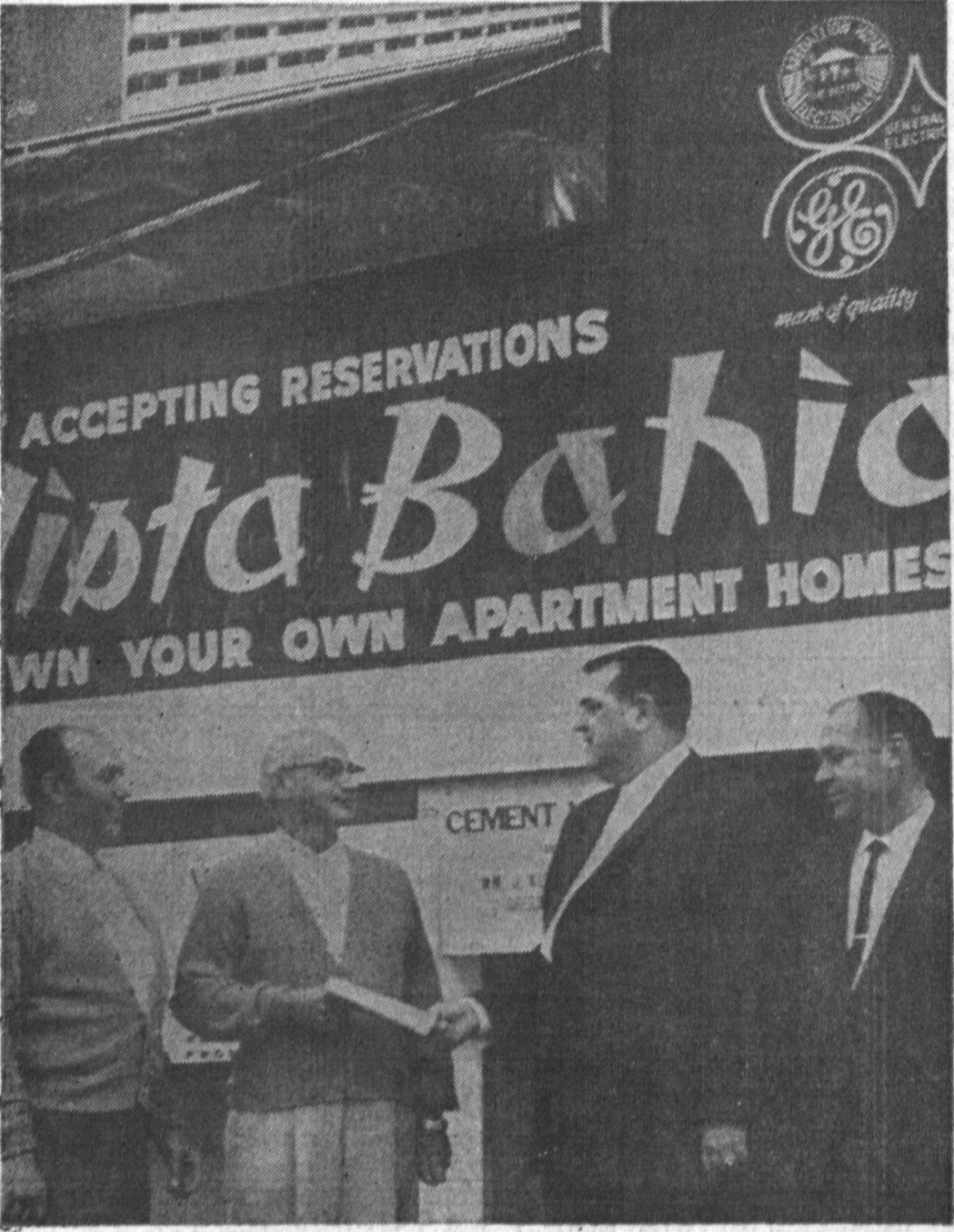
VISTA BAHIA own-your-own apartments near initial stages of construction at 201 Calle Miramar, Hollywood Riviera. Taking part in groundbreaking are (l-r) George Dighera, vice-
