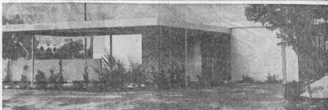
DISTINCTIVE —Three distinctive roof treatments have been designed for first models of the new Rheemetal home. A flat roof, as shown in this model, blends with its desert setting at Palm Springs. The structural system used in Rheem Manufacturing Company's new steel home is a direct translation of a system used successfully by its Rheemetal Building Division in con-
