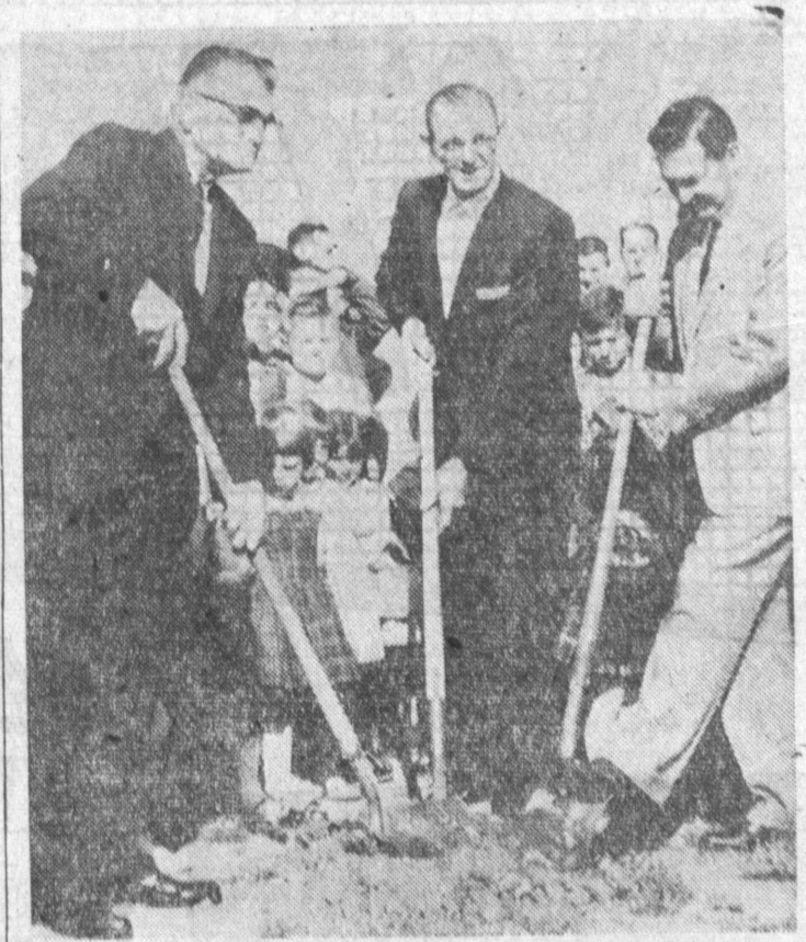
EDUCATIONAL BUILDING —Ground breaking for the new educational building construction started by members of the Calvary Baptist Church, 23601 South Main St., North Wilmington, was held last week. Turning the first soil are Pastor Irwin, John Clark, chairman of the board of trustees, and Herman Trimm, new building chairman. Sunday school is at 9:30 a.m., morning worship service is at 11 a.m. and BYF meets at 6 for teenagers, and 6:30 p.m. for college and young married people.
