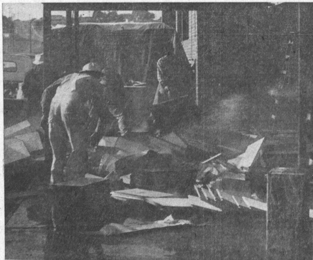
SOUTH HIGH SCHOOL FIRE —Forty cases of acoustic tile lay in a smoldering heap today, the aftermath of a fire Thursday at South High School's new addition, under construction. Started by a spark from a welding torch, the fire also destroyed a paint-
