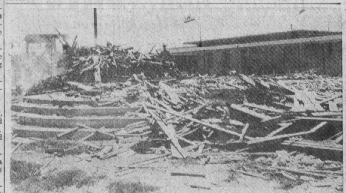
SCHOOL HOUSE TOPPLES — The front steps are all that remains of the old administration building of the Perry Elementary School 184th St. and Prairie Ave. Constructed in 1924, the old building has been replaced by classrooms at the Madison Elementary School. Remainder of Perry campus has been built up in last few years.
