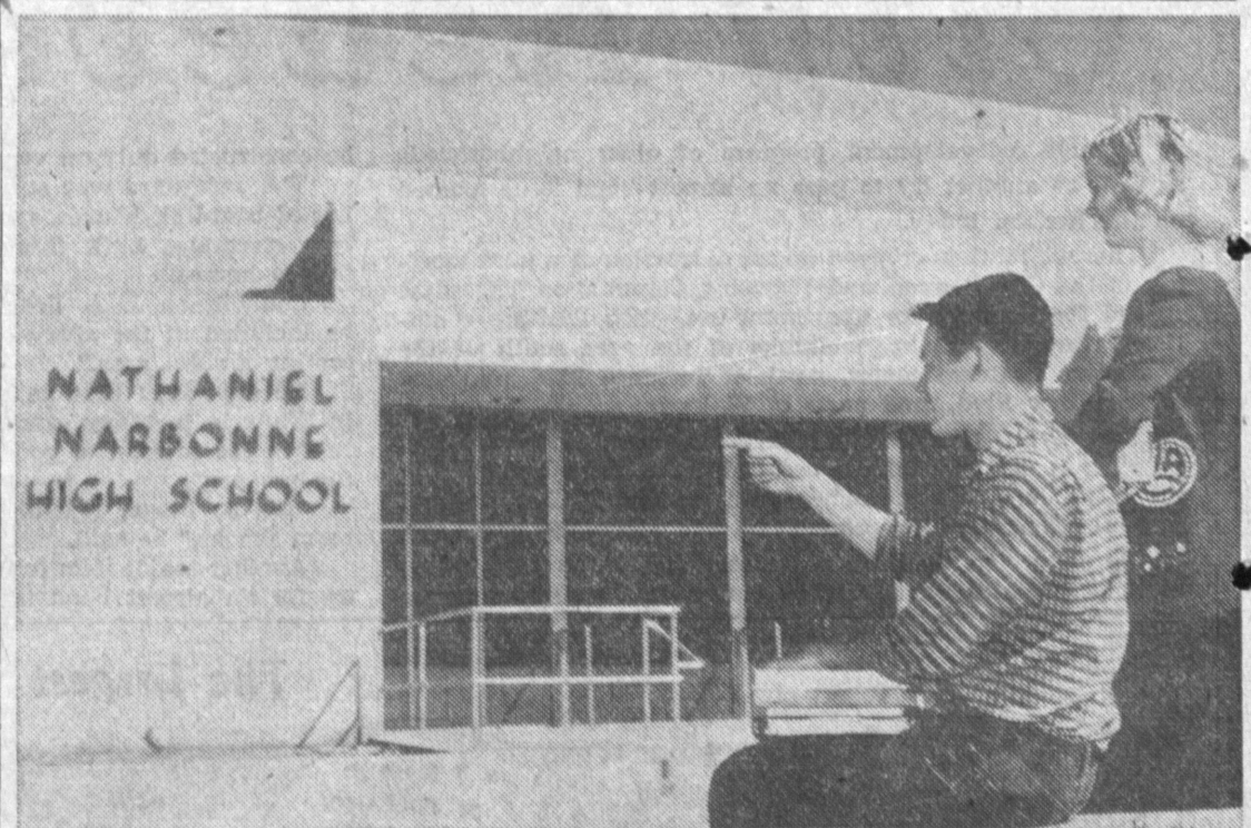
NEW AUDITORIUM — Seniors Pete Neushul and Janice Cook relax in front of new 1000-seat auditorium at Narbonne High School at 24300 S. Western Ave., which was dedicated Friday night. The building, which combines the latest innovations in equipment, cost a total of $422,000.
