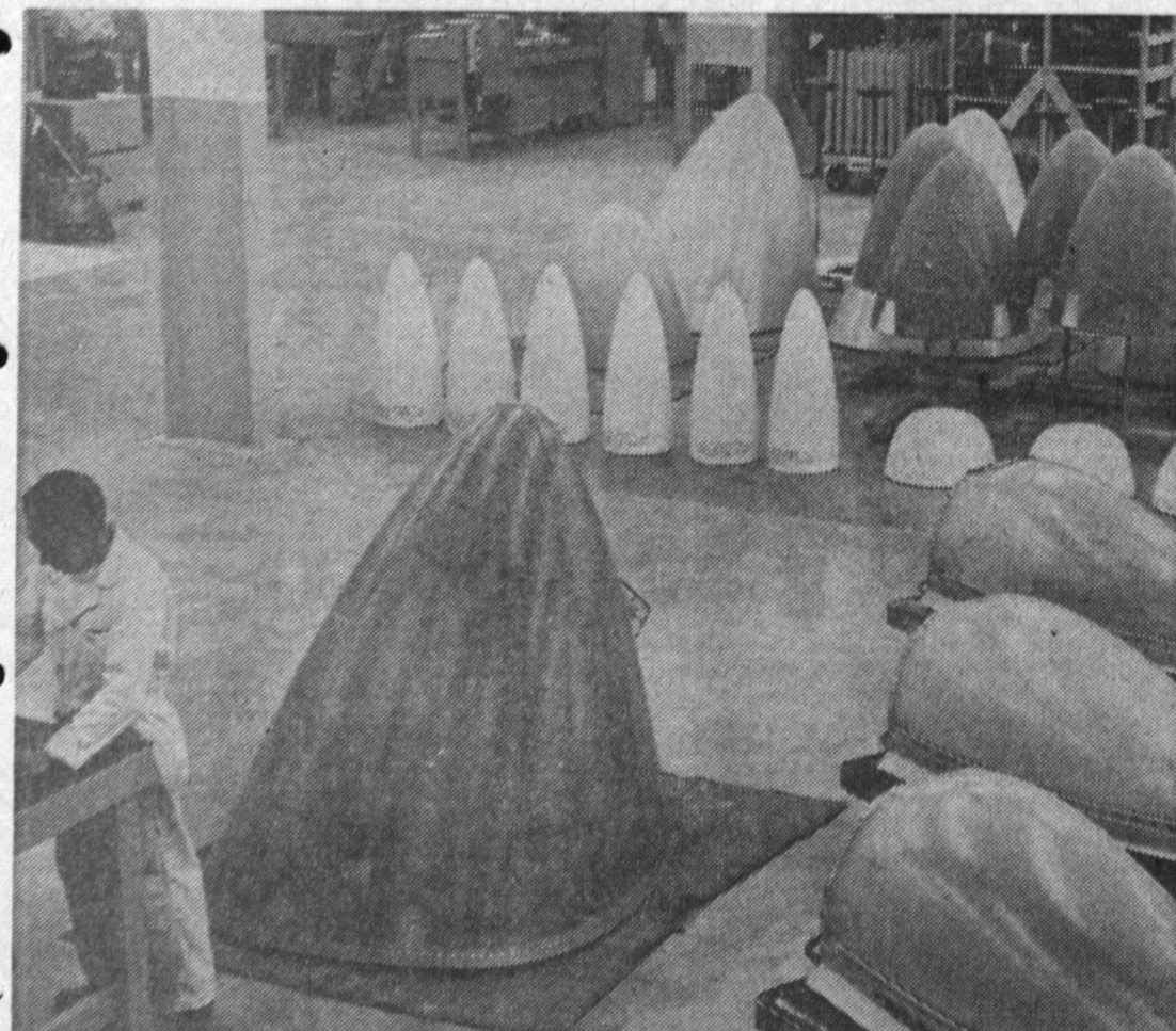
PAINT DEPARTMENT — Completed radomes, just a few of the many plastic products manufactured at the Douglas El Segundo Torrance facility, receive outer coating of paint in three major paint booths.
