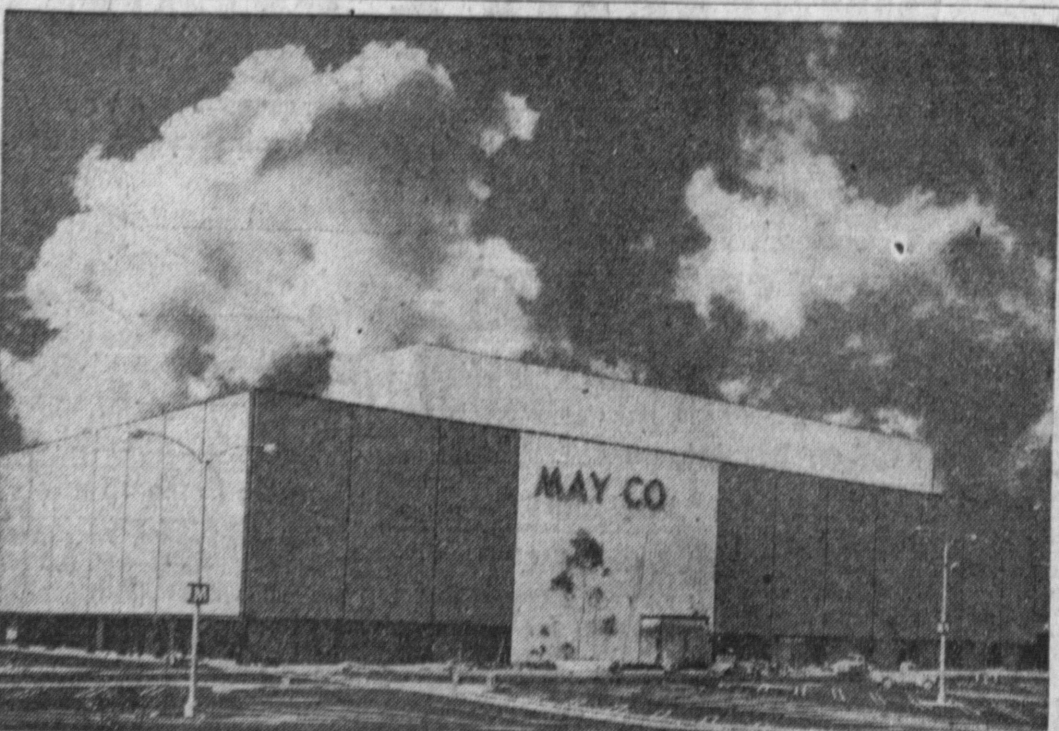
OPENS MONDAY—The new South Bay May Co. will open Monday in the South Bay Shopping Center, Hawthorne Blvd. and 174th St. The modern new store will have three floors and contain 351,000 square feet of floor space. (More pictures on page 8)
