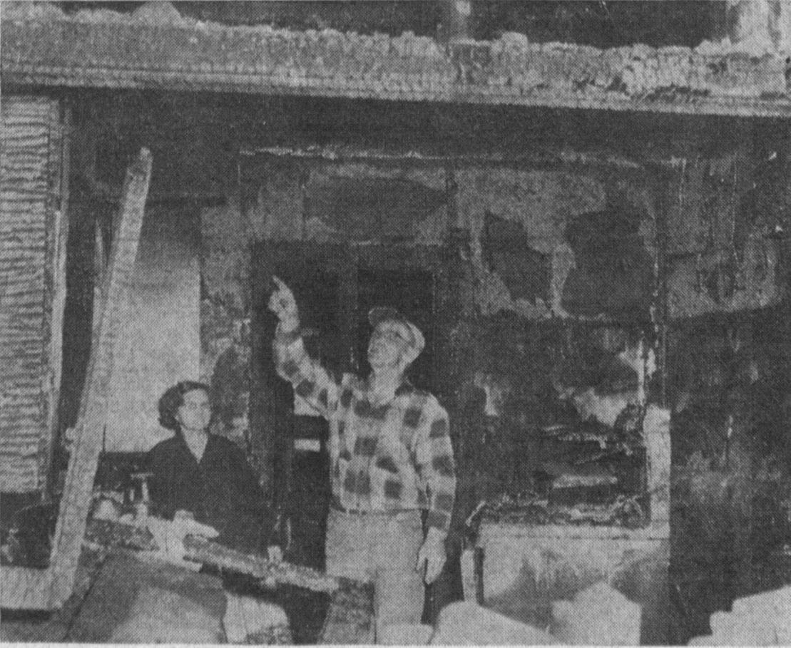
FIRE DAMAGE —Mr. and Mrs. William Howell, inspect the home of Mrs. Marguerite Givens, who claims that low water pressure in the South Torrance area, caused delays in fighting the fire. Firemen admit it took several minutes to boost pressure to an effective level. Press Photo.
