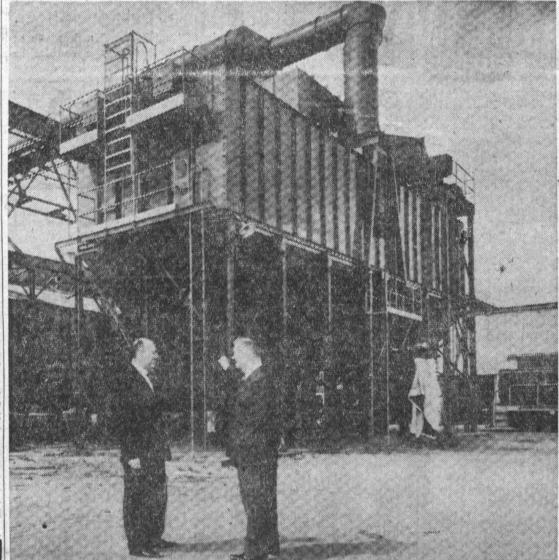
NATIONAL SUPPLY COMPANY'S four room "baghouse" is shown by National's works man-ager J. D. Spalding to Torrance Mayor Albert Isen. The baghouse is actually a huge vacuum cleaner which carries dust particles from the plant to large bags in the new structure. Ducts over the electric melting furnaces carry all smoke to the baghouse. The dust particles are
