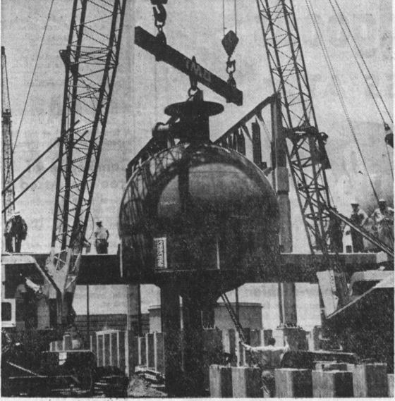
One of three spherical reactors at the new catalytic reformer being built at General Petroleum Corporation's Torrance refinery is raised by two cranes for setting on foundations. Each reactor is about 20 feet high and weighs 100,000 pounds. These
