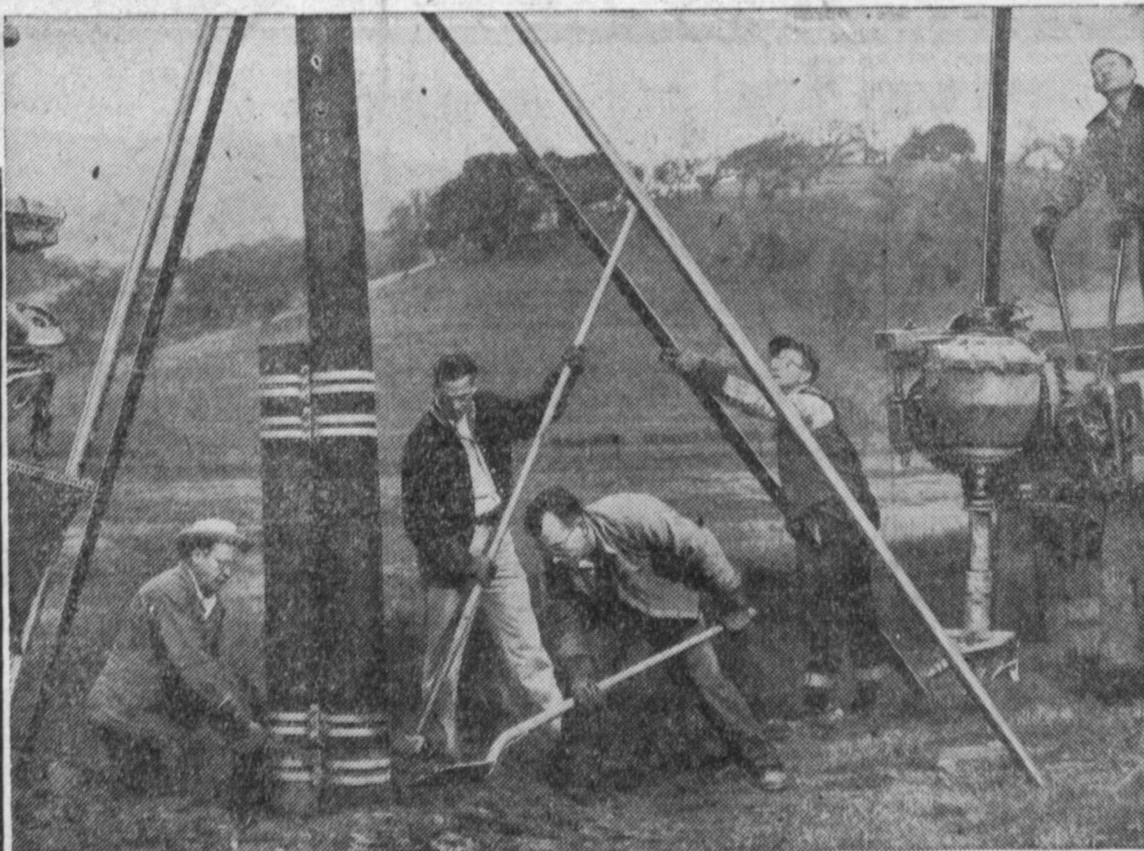
"Pole stubbers" at work: Inspection has revealed a pole which shows damage at the ground line. Now, reinforced with a short length, it will be strong as new, and we'll have saved much of the cost of a new pole.
