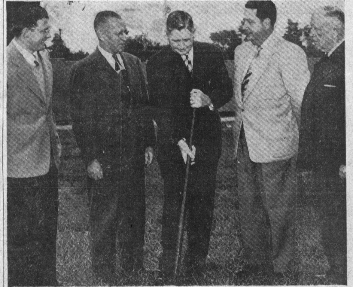
TORRANCE MAYOR — Bob Haggard turns the first spadeful of dirt at informal ground-breaking ceremonies held this week to launch the start of construction work on Pacific Telephone's new dial center at the southeast corner of Cravens and Engracia avenues. Others present (left to right) included: William Zappas, of the Torrance Press; A. B. Smith, telephone manager; F. Y. Snyder, district telephone manager; and Blaine Walker, executive secretary of the Torrance Chamber of Commerce.
