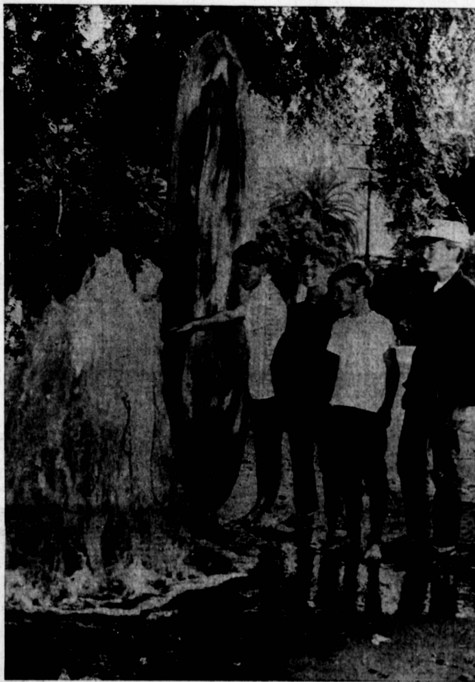
SURFIN' WEATHER... Four El Nido area lads check the surf in the street in front of 18319 Mansel Ave. after a city trash truck broke through the paving and snapped a high-pressure water line. With the surfboard is Gene Thomas, who is backed up by Gary Jackman, Steve Thomas, and Ward Miller. The boys decided to wait for better waves. (Press-Herald Photo)
