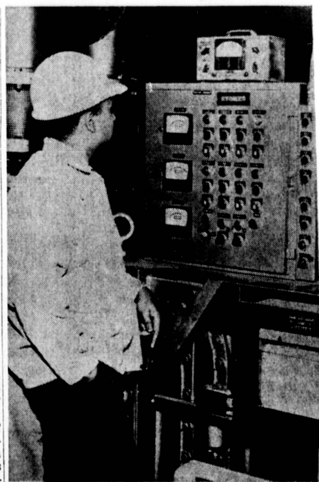
CONTROL PANEL . . . A workman at the Torrance facility of National Supply, a division of Armco Steel Corp., takes a look at the control panel for a new vacuum degassing steelmaking process now being used in the Torrance plant. The process produces stronger, cleaner, and more uniform steel by removing hydrogen gas from the molten metal as it is poured into a special airless chamber.
