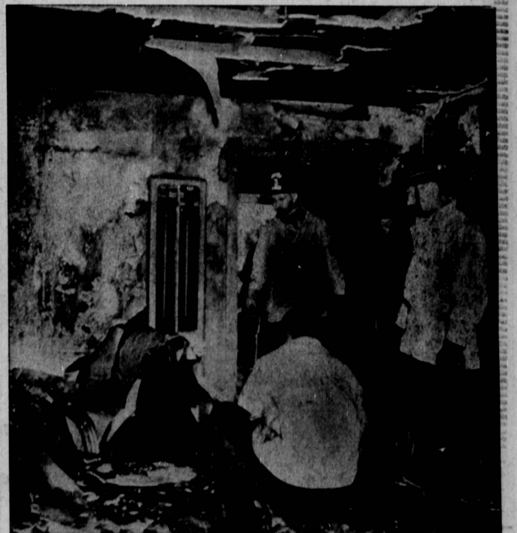
GUTTED HOME . . . Firemen probe the ruins of the home of Mr. and Mrs. Rhodes Radar at 18528 Grevilla Ave after bringing the blaze under control Thursday morning. The home was totally destroyed and most of the family's personal possessions were turned to smoke. The family dog was killed in the blaze, but Mr. and Mrs. Radar and their six children were not at home when the fire broke out. (Herald Photo)
