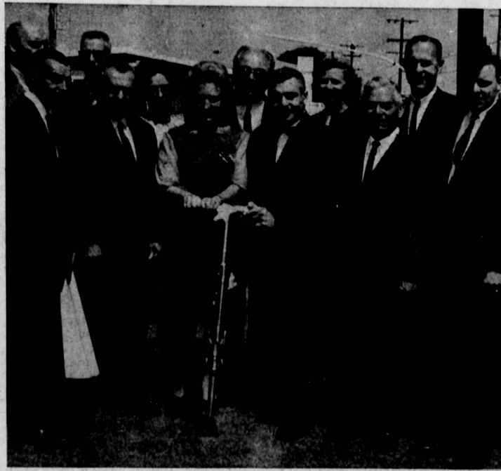
FOR NEW LIBRARY . . . Ground breaking ceremonies for the $82,000 North Torrance Library were held yesterday just before noon. Pictured around the air hammer used to break through the parking lot at the site are: Weldon Fulton, architect; Councilman Ross Sciarrotta; Mrs. Claire Crain of the Library Commission; City Manager Ed Ferraro; Councilman Victor E. Benstead Jr.; and city librarian Harold Umberger. Others are J. L. Rea, Councilman J. A. Beasley, Lee Addison, regional librarian, Councilman Nicholas Drale, Mrs. W. L. Saville, and Councilman Ken Miller. (Herald Photo)
