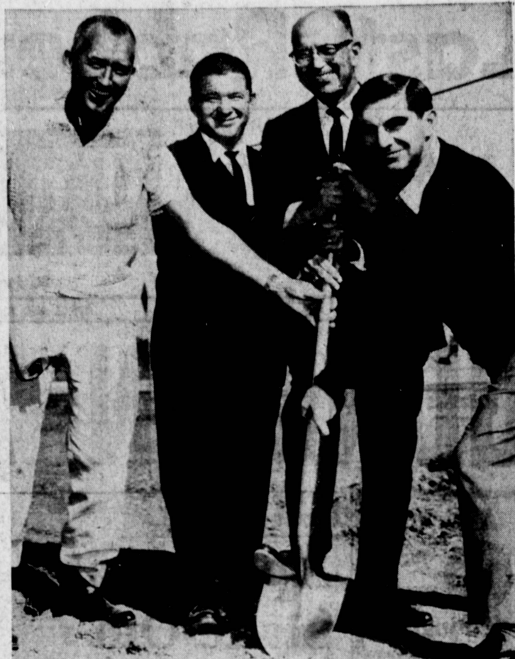
FOR NEW STORES . . . Ground breaking ceremonies for a $500,000 addition to the Rolling Hills Plaza shopping center were held Thursday morning with Mayor Albert Ison officiating. The new building activity will add 18 new stores to the center and provide parking for 240 more cars.
