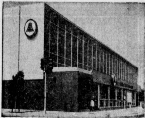
INFORMATION SERVICE . . . Will be provided from this ultra-modern building at 2154 Torrance Blvd. starting Sunday. Thirty-six switchboards will be open daily to provide local "113" data regarding Pacific Telephone subscribers in Torrance, Gardena, Wilmington, Lomita, San Pedro, and a portion of Compton.
