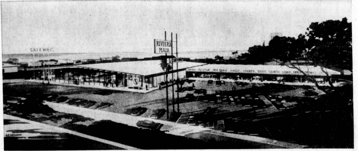
RIVIERA PLAZA STARTED . . . An ultramodern Safeway Store will be the key commercial facility in the new Riviera Plaza Shopping Center now under construction by Ernest W. Hahn, Inc., in Hollywood Riviera. Developer of the project is Paul O'Kane. Completion is scheduled for July.
