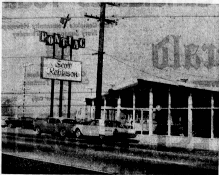
TORRANCE NEWCOMER . . . Scott Robinson Pontiac's new sales and service facilities at 20340 Hawthorne Blvd. features both new and used cars. Their service garage boasts of having the best mechanics. (Herald Photo)
