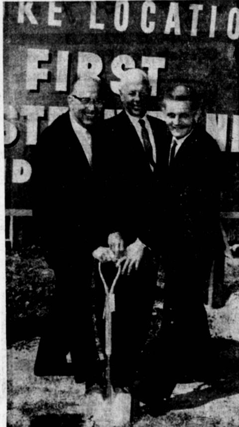
BANK STARTED... Ground for new 7,458 sq. ft. facility for the First Western Bank & Trust Co. at 23865 Hawthorne Blvd., was broken Friday in ceremonies attended by bank and civic officials. Here Mayor Albert Isen (left) helps J. Arthur Taylor, chairman of the board, and Ed Talbot, manager, with the first shovel of earth. (Herald Photo)
