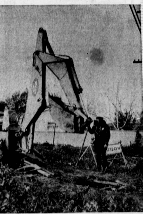
POSSIBLE TRAGEDY AVERTED . . . Torrance Police Department Motorcycle Officer Ken Halbert stands by while a city tractor fills a 6 1/2-foot-deep hole on a pie-shaped lot where Calle Miramar, Via Colusa and Paseo De Arena merge. The hole had apparently been dug by children and covered with scrap boards. The site is near Riviera Elementary School. (Herald Photo)
