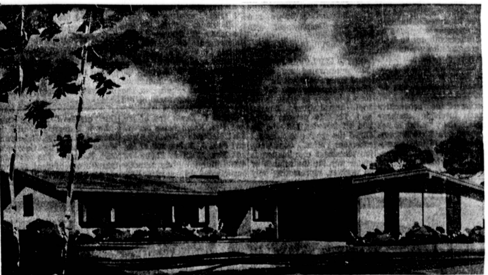
FAST-SELLING PENINSULA HOMES . . . Shown is one of the varied stylings at The Estates, new Grandview Palos Verdes development priced from $25,550, with monthly payments from only $146. Spacious homes include wall-to-wall carpeting, custom-styled fireplace, built-in kitchen appliances.
