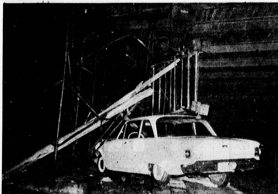
SUPPORTS TOPPLED... Crews working on the San Diego Freeway in Torrance were called out about midnight Sunday to replace temporary bridge supports on Crenshaw overcrossing after this auto, driven by William Henry Volmerding, 48, of 2083 Middlebrook Road, slammed into
