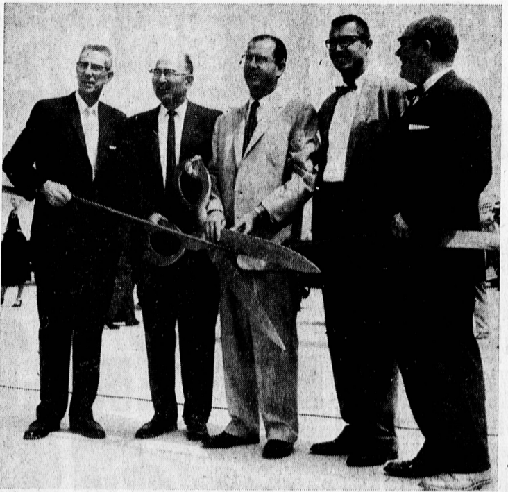
TORRANCE OFFICIALS . . . Joining in ribbon-cutting to open new link of Harbor freeway are (from left) Councilman J. A. Beasley, Mayor Albert Isen, Supervisor Kenneth Hahn, Public Works Director Wade Peebles, and Councilman Nickolas Drale.
