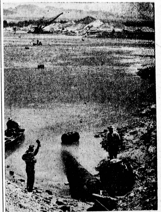
ACROSS THE RIVER . . . Workman signals as pipeline is pulled from the Colorado river in completion of the first underwater river crossing to provide out of state natural gas for customers of Southern California and Southern Counties Gas Cos. The 1458 feet of pipe was dragged across the river by two 1 1/4-inch cables attached to a huge winch.
