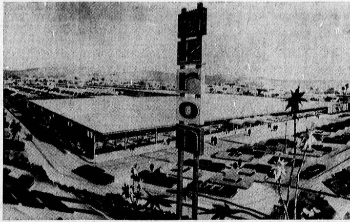
OPENING NEXT WEEK . . . The huge new Akron at Hawthorne Blvd. and 180th St. will open next Tuesday, March 29, at 9 a.m., it was announced here this week. The new facility will provide every shopping convenience for The growing Torrance-South Bay area, including ample off-street parking.
