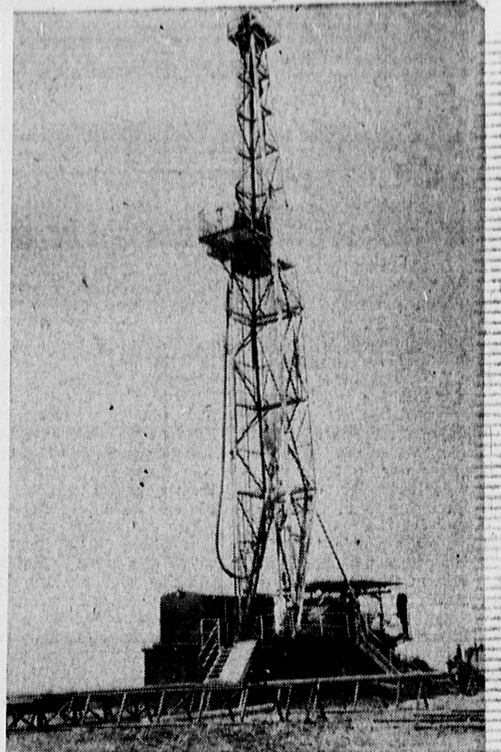
VETERAN RIG . . . This drilling rig, owned by Brinkhoff Drilling Company, Denver, has been used to drill 159 wells, with a total of 849,251 feet, in a little over four years. It is a skid-mounted National T-20, manufactured by The National Supply Company, powered by GMC Twin Diesel Engines, and includes a 95-foot Lee C. Moore Mast. The record averages about 38 wells, of 5,341 feet, each year. Normally the rig is transported in ten loads.
