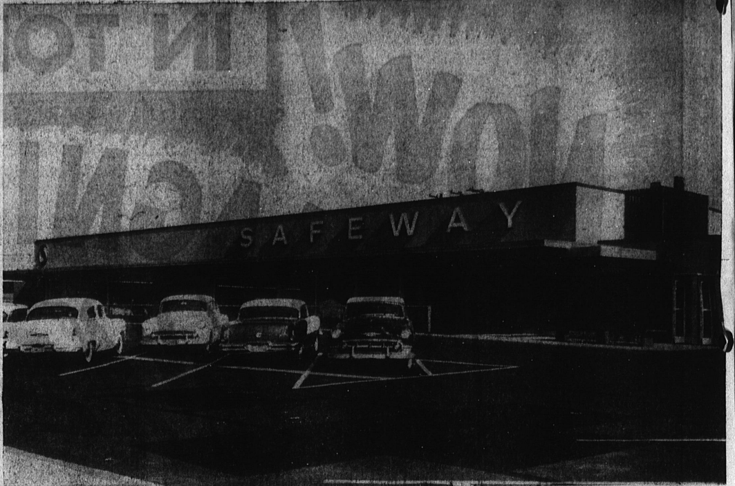
PLENTY OF PARKING... The new Safeway Store at Carson and Western Ave. features plenty of easy-to-reach parking. Wide parking stalls, reached through ample traffic aisles, make the problems of parking
