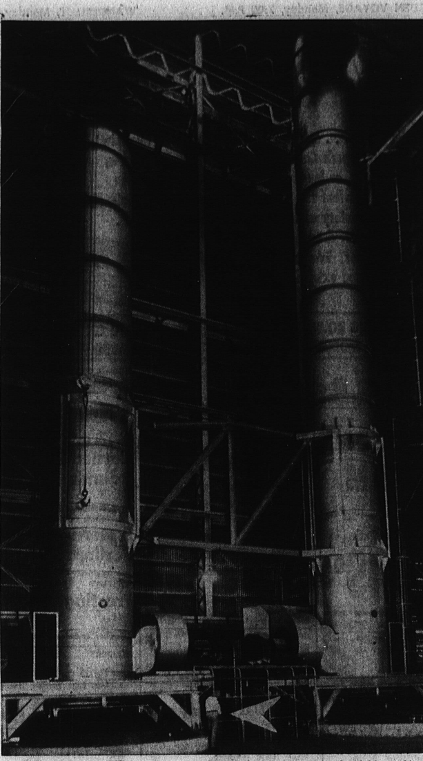
TEN-STORY FURNACE... The nation's largest electric furnace on the right, reaching higher than a 10-story building, treats giant aluminum alloy shapes for various uses at the Harvey Aluminum plant here.
