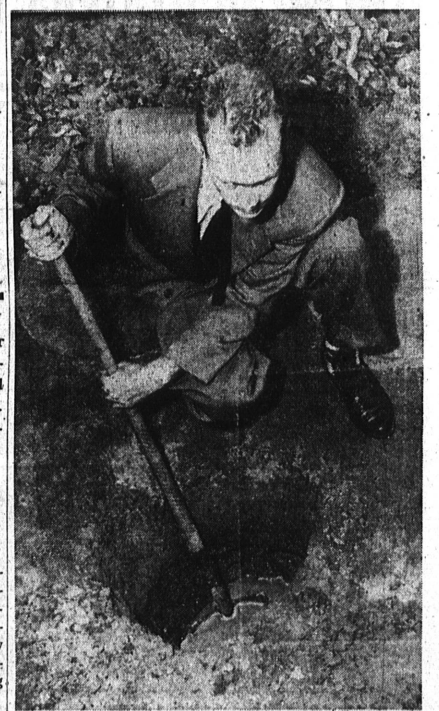
CHECKS WATER FLOW . . . James Post, 3118 Sonoma Ave., check flow of water into hole dug in back yard of neighbor Glen Keller, 3114 Sonoma, as residents become alarmed at the situation. Engineers say improper drainage may be causing water to accumulate in the back yards of half a dozen Sonoma Ave. residents.
