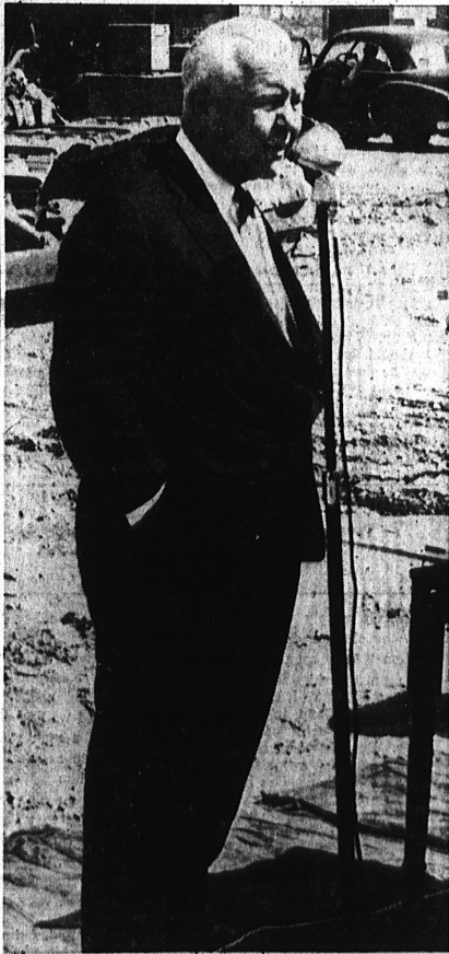
PLEDGES COOPERATION . . . Walter J. Bruemark, vice president and general manager of the May Co. Los Angeles, told those at the groundbreaking ceremonies this week that his company didn't want to move in and re-write the rules for the area. "We want to become a part of your community and operate by your rules," he said.
