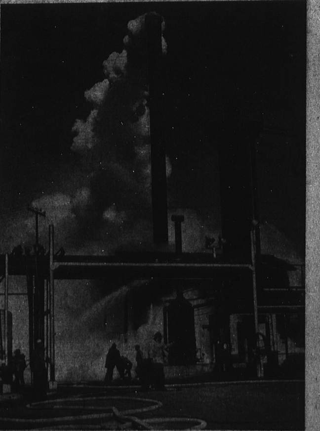
AT HEIGHT OF BLAZE . . . Firemen from eight companies battled flames at Sunset Oil's Torrance refinery Sunday afternoon after a fuel line ruptured on one of the plant's heating units. Here fire fighters pour water into unit to control flames shortly after fire broke out. Men of Co. 36 on Carson St. heard the explosion, reported to the fire immediately.
