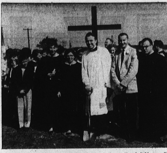
GROUND BREAKING RITES . . . Christ the King Lutheran Church held groundbreaking ceremonies for its new church at 2706 W. 182nd St. last Sunday. The new structure is expected to be ready by early summer. Taking part in the ceremonies were Robert Jones, Sunday school; Ora Denney, Luther League; Mrs. Elton Crump, church women; the Rev. Maynard Midthun, pastor; Bill Sands, board of trustees, and Mike Bankson, board of deacons. Special music was presented by the choir.
