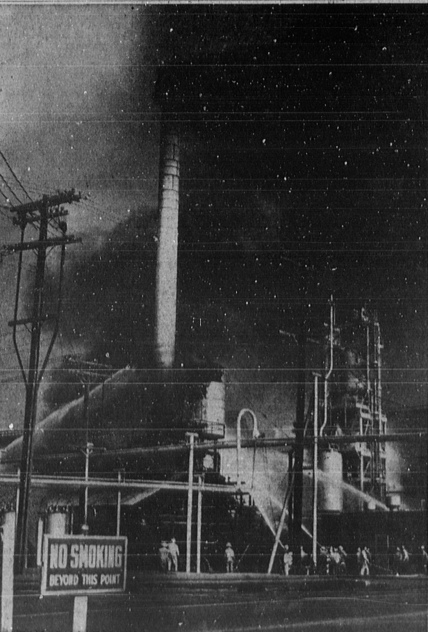
FIREMEN BATTLE OIL BLAZE . . . Torrancia and General Petroleum firemen join forces to battle raging oil fed fire at the Torrancia refinery Thursday morning. A ruptured pressure line in the visbreaking unit caused a jarring explosion which nearby workers described as "sounding like a bomb."
