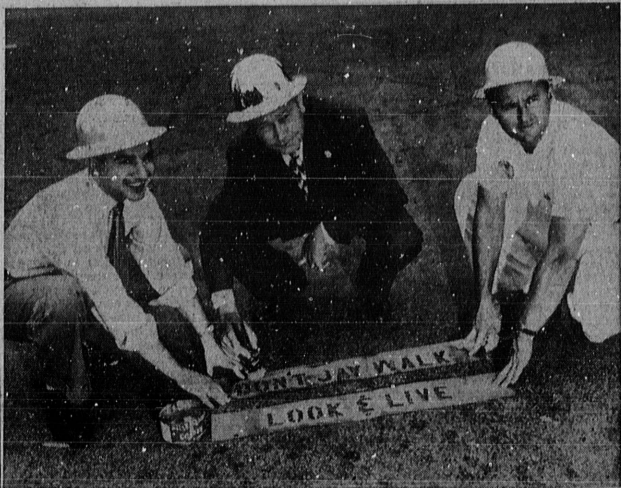
A DRIVE FOR SAFETY . . . Another 1950 project of the Junior Chamber of Commerce in Torrance was the safety campaign which was kicked off when members of the service organization painted safety reminders on street corners, sidewalks, and other spots throughout the city which could be a safety hazard. Here former Mayor Bob Haggard (center) helps two Jaycee members paint one of the city's streets with the slogan "DON'T JAYWALK—LOOK & LIVE."
