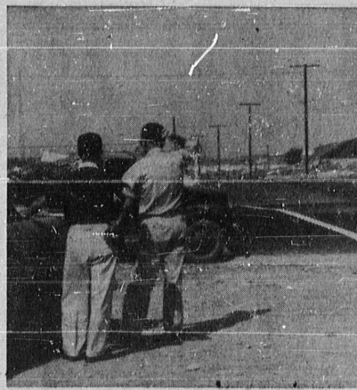
WATCHING TRAFFIC . . . Two representatives of the traffic division of the Department of Highways watch the flow of traffic past 230th and Hawthorne Blvd. Friday, as part of a check on conditions there. The check followed protests of mothers of Meadow Park School children, who are demanding yellow crosswalks or a stop signal.
