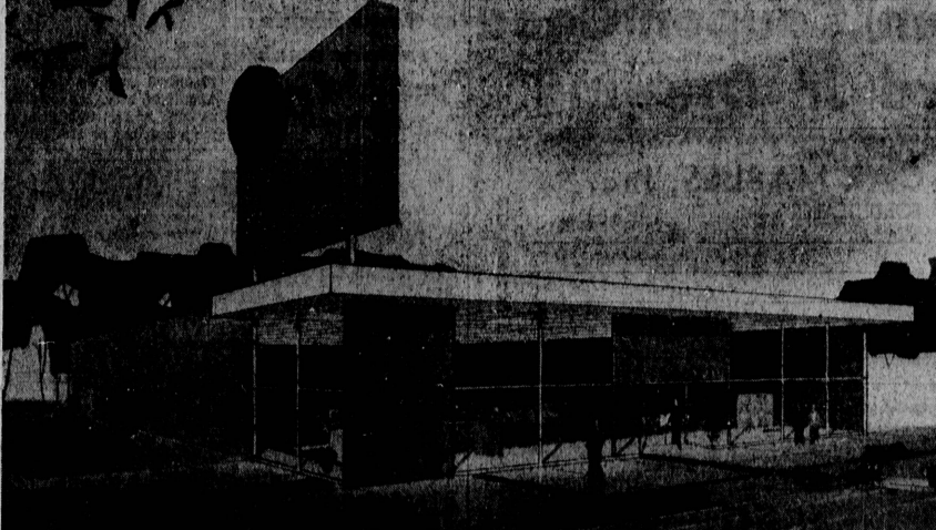
Our New Home Now Under Construction at 135th & Hawthorne Blvd.
