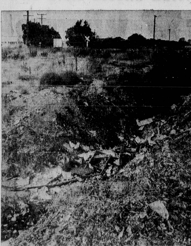
DUGOUT . . . This huge hole in the ground will be one of many problems facing fathers of Little League and Babe Ruth baseball players this winter when they begin leveling and grading land formerly used as a city dump at Plaza del Amo and Border Ave. for use as two Little League and one Babe Ruth diamond for next season's play. The city recently leased the leagues the land for five years for $5. View is toward Western Ave. Labor and materials for the huge job will be mostly donated by generous Torrance citizens.
