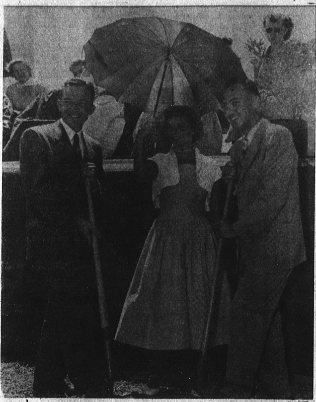
FIRST STEP . . . A long, hard struggle came to a gratifying climax recently when the ground was officially broken to start the construction of the new Watteria Community Methodist Church. Shown welding shovels in the shade are the Rev. Gene M. Gehres, left, pastor; Robert S. Cramer, right, chairman of the church building council, and Janet Van Dyke, holding umbrella. Over, 150 members of the congregation gathered to watch the ground-breaking. Speakers included Cramer, M. M. Schwab, Nate Gordon, the Rev. Douglas Walters, Buell Thomas, and the Rev. Harry McFarland. A potluck dinner followed the ceremony.
