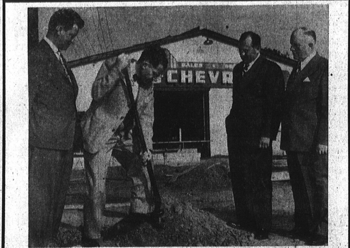
JUNE 14, 1947 — Paul Loranger, owner, watches while Mayor J. Hugh Sherkey Jr. turns the first shovelful of dirt for new building. Watching the ground-breaking are Gus Culbertson, (second from right), then zone manager for Chevrolet; and (right) Chamber of Commerce Secretary Blaine Walker.
