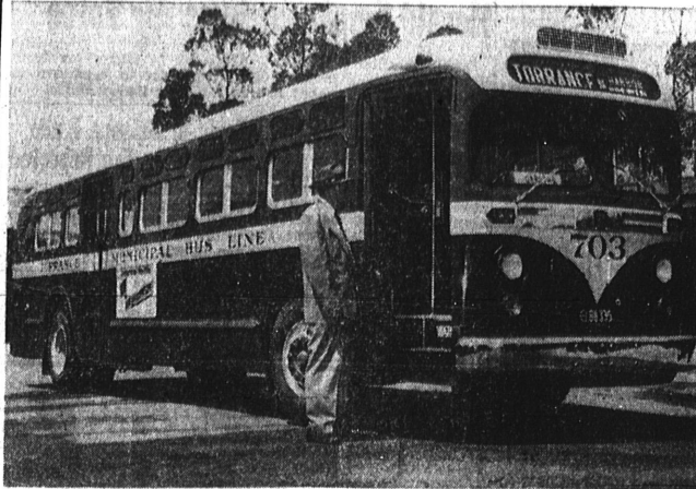
RIDING ON AIR . . . Bus Superintendent Marshall Chamberlain looks over the city's new bus which went into service here this week with the amazing new "riding on air" feature. The 45 passenger bus has a series of heavy air bellows on which the body rides, and without springs, shocks, and other "metal on metal" parts, the maximum reduction of squeaks and other noises is eliminated.
