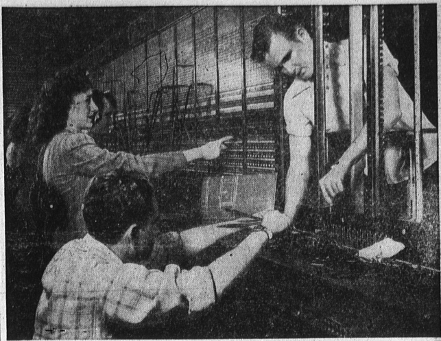
Many skills of many people go into the big job of providing telephone service in the West today.
